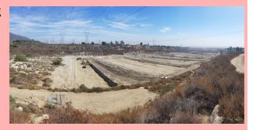
Holly Drive Booster – Construction of the new water pump building is wrapping up. This new pump house will deliver more water more efficiently to the Holly Drive reservoir site. This project improves fire protection and will work in conjunction with the new 120,000-gallon Holly Drive Reservoir scheduled for construction in 2019.
