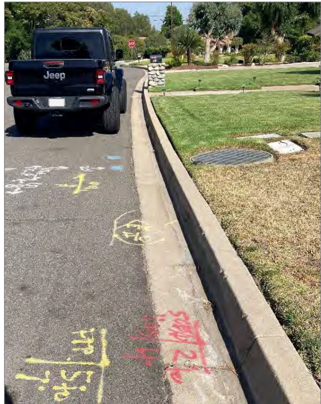
Figure 2 – Glendale Rd. facing east. Utility boxes in grass and USA markings on street.
