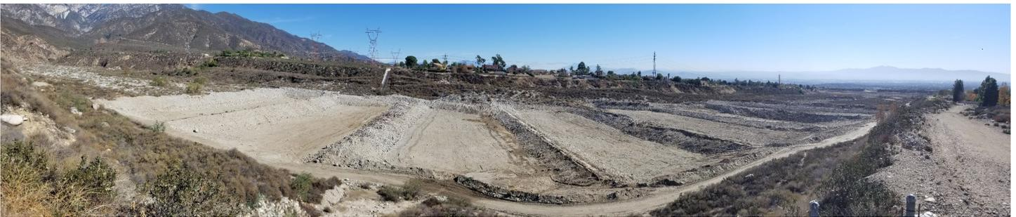
Above, the Crosswalls before the rain. Below, after the rain came in April 2020. Crosswalls working like they are designed to do which is to trap and store canyon flow, allowing it to percolate into and recharge the groundwater.
