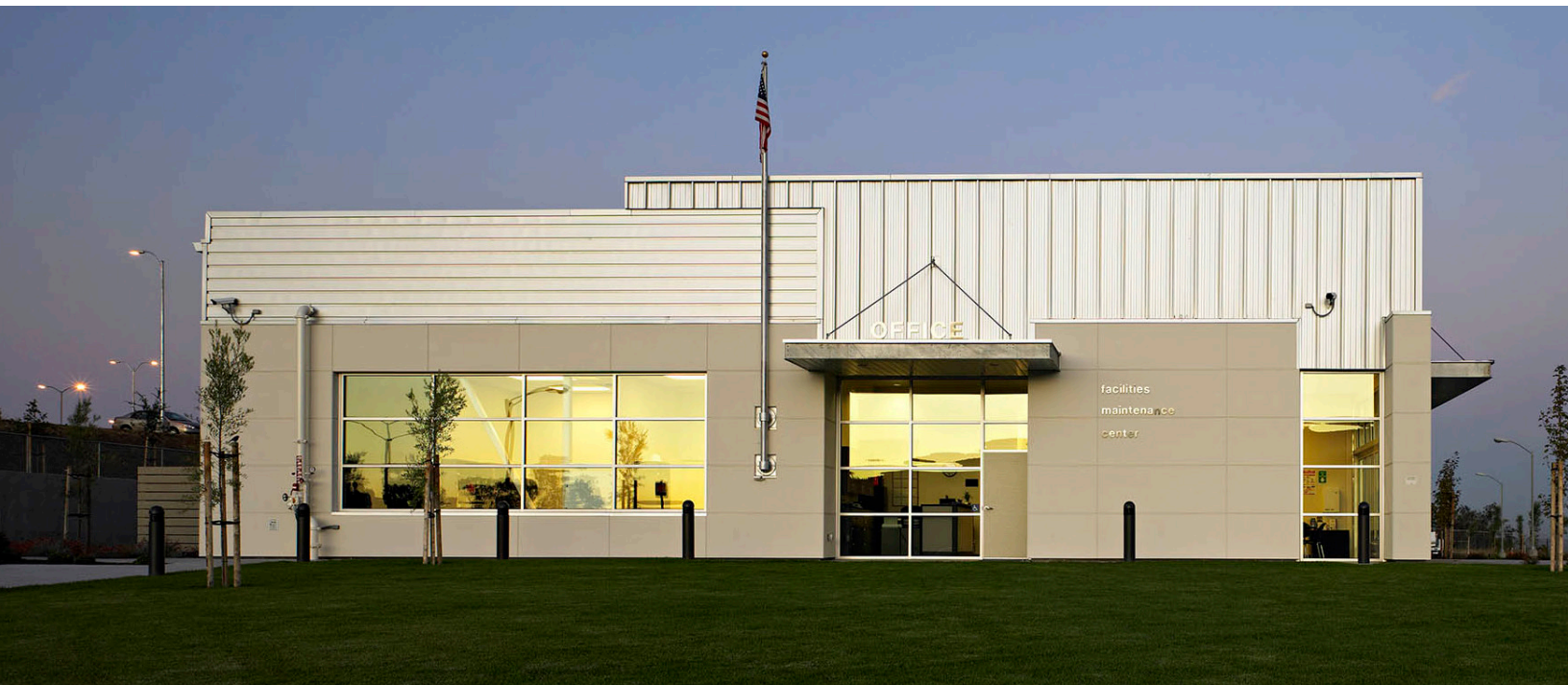
Facilities Maintenance Center at Cañada College | Redwood City, CA
