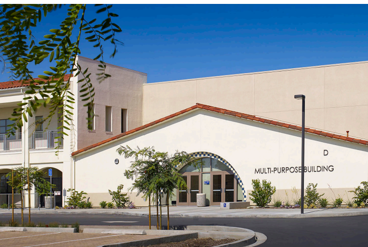
Marshall Elementary School (Mediterranean Architecture) | Anaheim, CA
